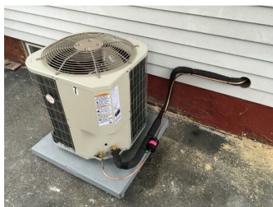
AC Refrigerant Line Insulation Missing
