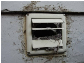
Broken/Clogged Vent
