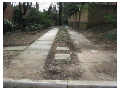
Erosion onto Sidewalk
