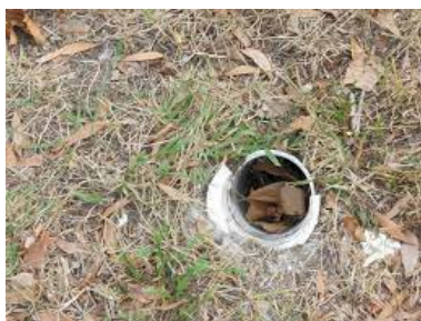
Missing Sewer Cap
