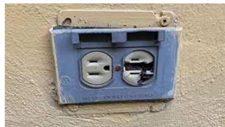
Damaged Outlet
